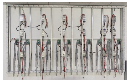
01 Install the frame and the power supply
